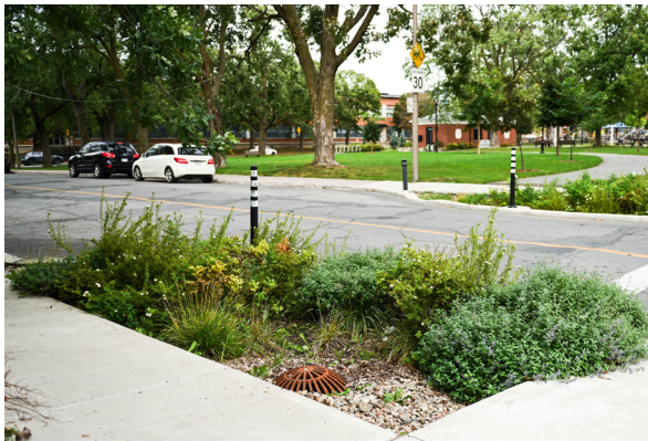
Figure 6. Standardized draining curb extension designed to retain and filter stormwater at street level
