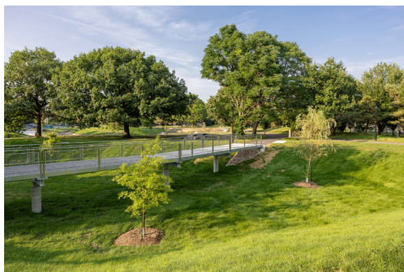
Figure 4. Overview of the Pierre-Bédard resilient park, designed to absorb and temporarily retain stormwater
